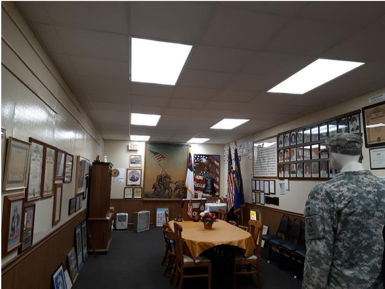
View of new ceiling & lighting, looking to the room front.
