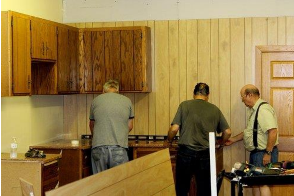
Construction Team sharing ideas, 7/24/2017.
