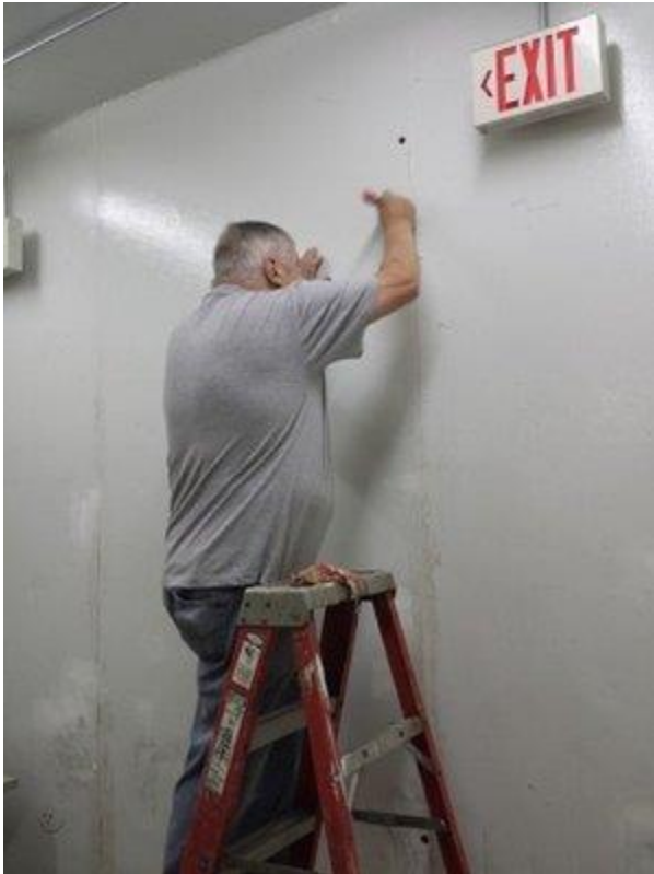
Jerry preparing the Post 501 History/Auxiliary meeting room wall for painting, 6/29/2017.
