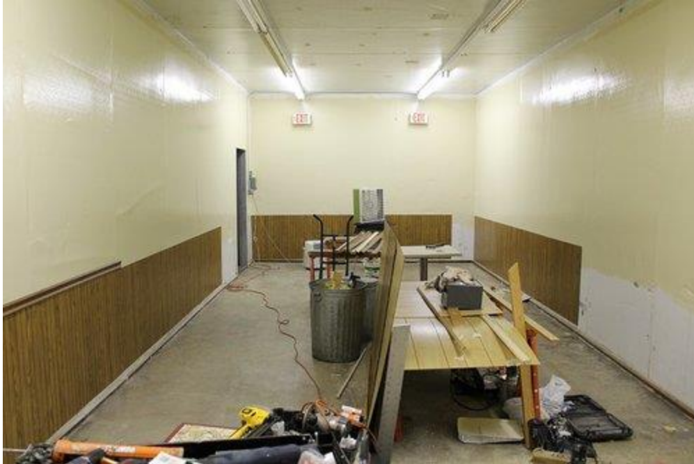
History/Auxiliary meeting room wainscoting installation in progress, 7/24/2017.
