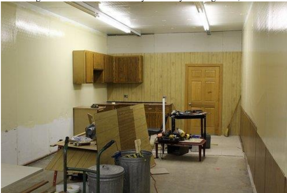
History/Auxiliary meeting room storage cupboards are installed, 7/24/2017.
